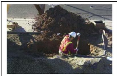
*Hand digging for telephone cables*
